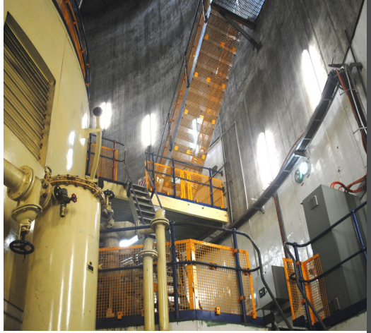
BLH Stop Drop™ Barricading installed on Stairways
