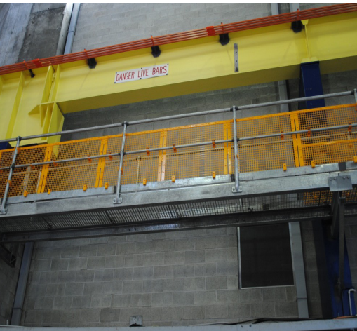
BLH Stop Drop™ Barricading installed on Walkways
